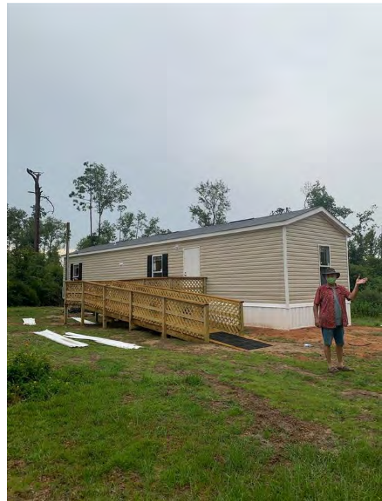
Figure 1: A recently completed mobile home placement in Altha, FL. This home has the addition of a new American Disability Act (ADA) compliant ramp to better accommodate the homeowner, whose mobility is limited.
