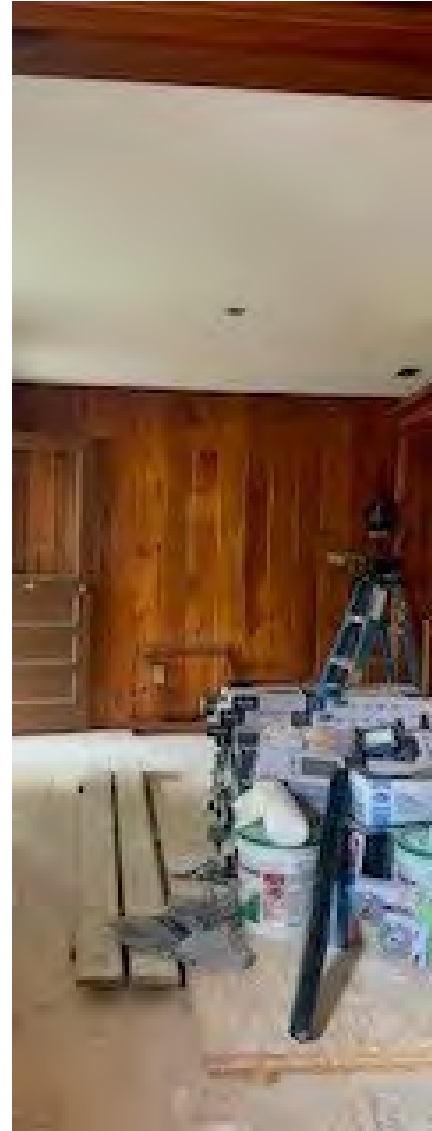
Fig. 1: Photo of rehabilitation project underway getting prepped for new flooring installation.
