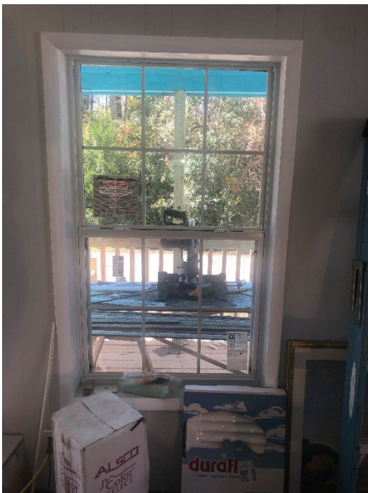
Figure 2: Installation of new windows throughout a residence.
