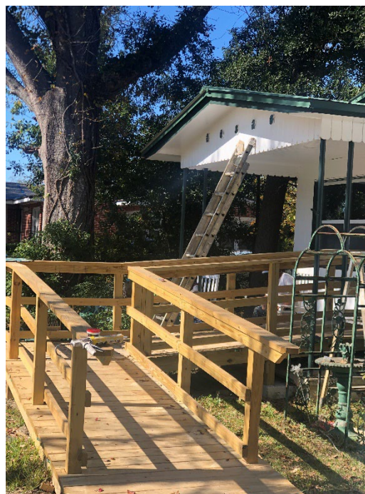
Figure 3: The addition of an ADA-compliant ramp added to a home.
