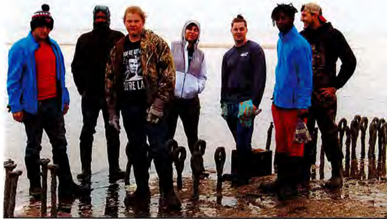
Environmental Planning Manager, Josh Adams (far right), works with members of the ED Corps, to install materials for the reefs at a test site for the Franklin-98 project.
